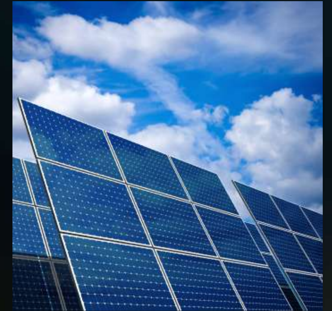
Typical PV panel array
