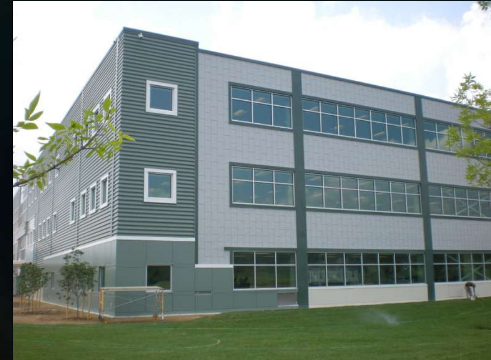
Current metal panel curtain wall system
