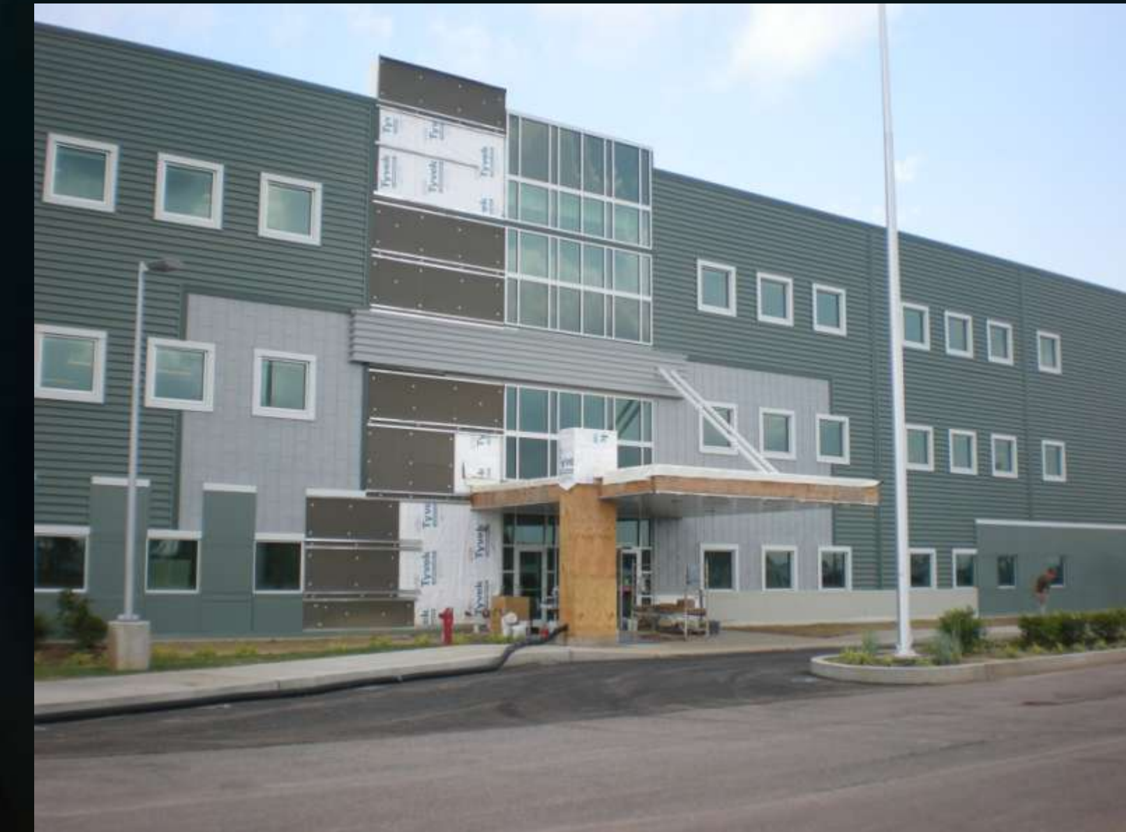
Missing panels on front façade of building
