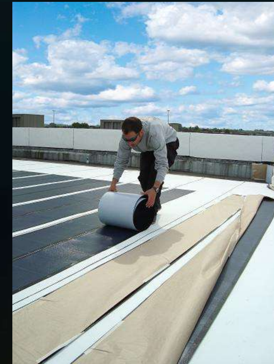
Installation of Uni-Solar panels
