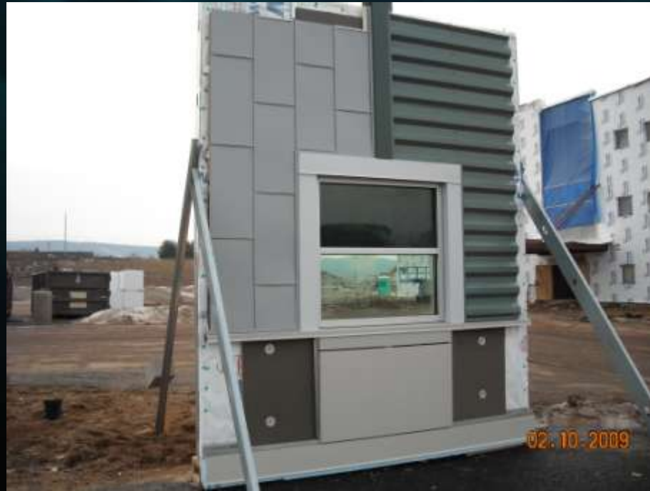
Curtain wall mock-up panel
