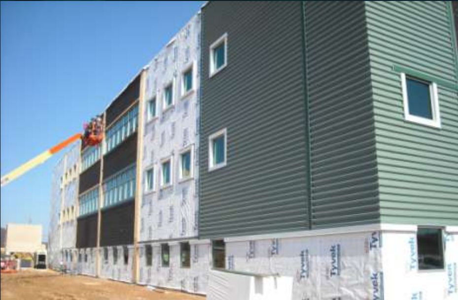
Construction of the curtain wall system
