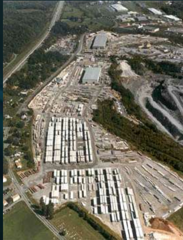
High's facilities – Denver, PA
